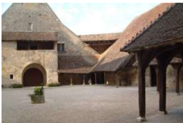
The main courtyard
